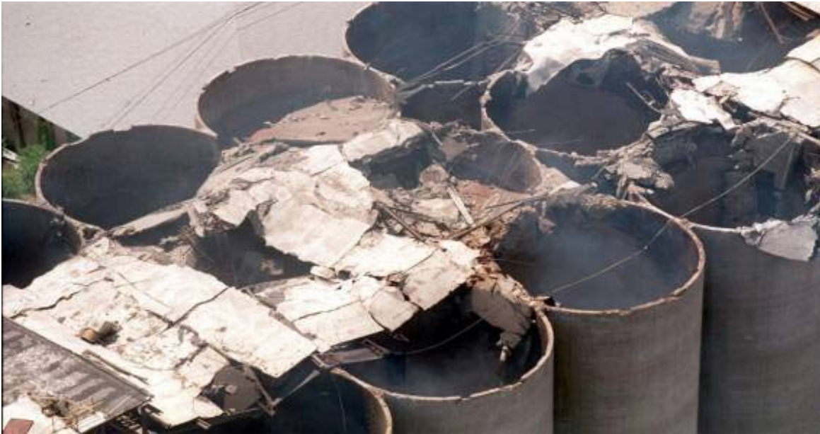
DeBruce Grain Explosion, OSHA Report
